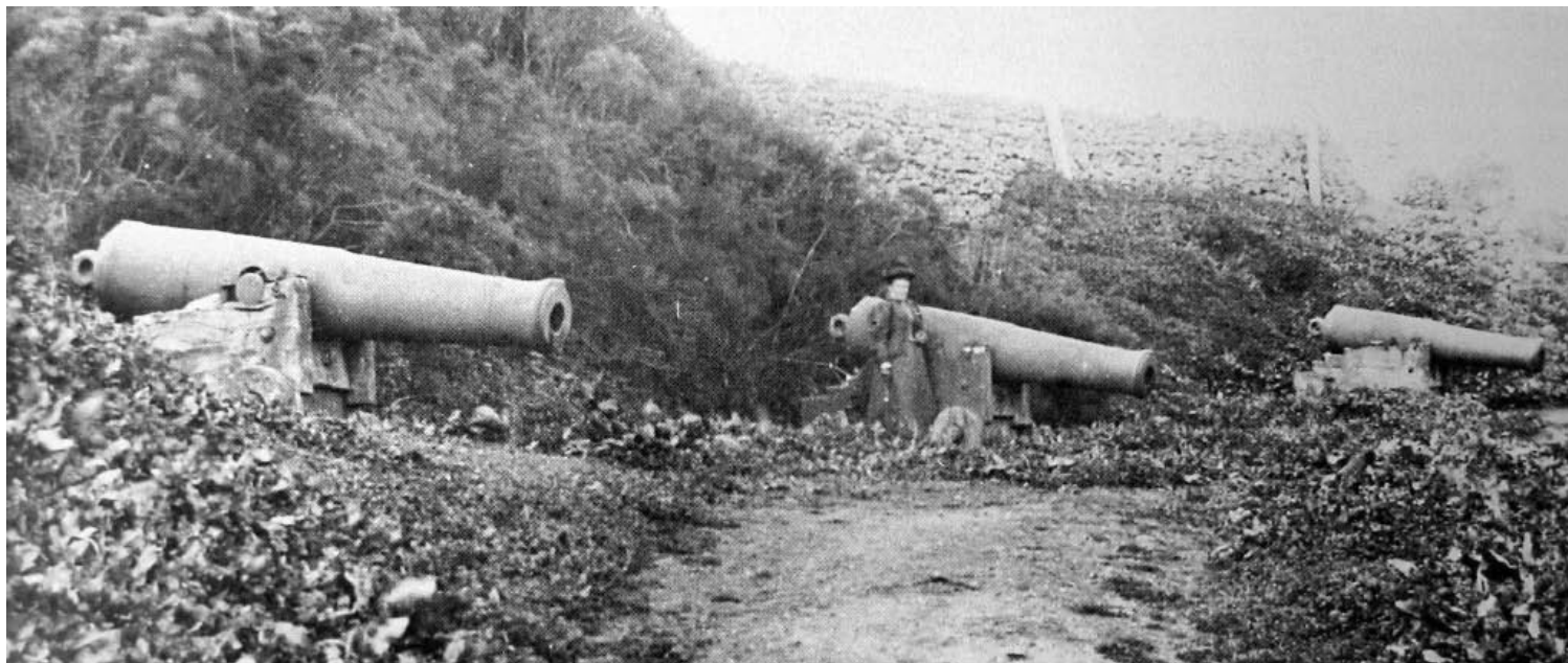
71cwt 64pdr Palliser Rifled Muzzle Loading Guns mounted on wooden Sea Service Carriages at Mt Victoria, Wellington, c1893.
