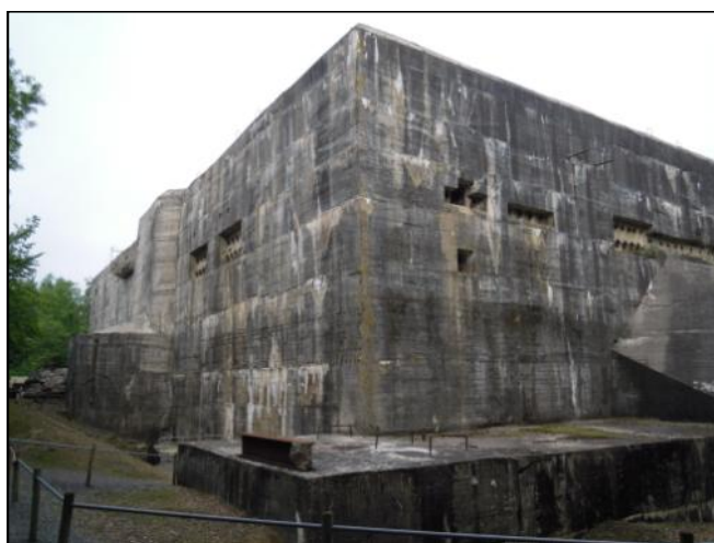
The massive concrete Block House where V2 rockets were assembled. Much of the surrounding land has been built up by several metres to allow easy access.
