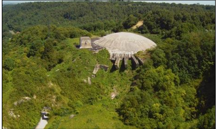
La Coupole from the air. Notice the dislodged concrete abutments caused by bombs and the tunnel entrance at the bottom left hand side.
