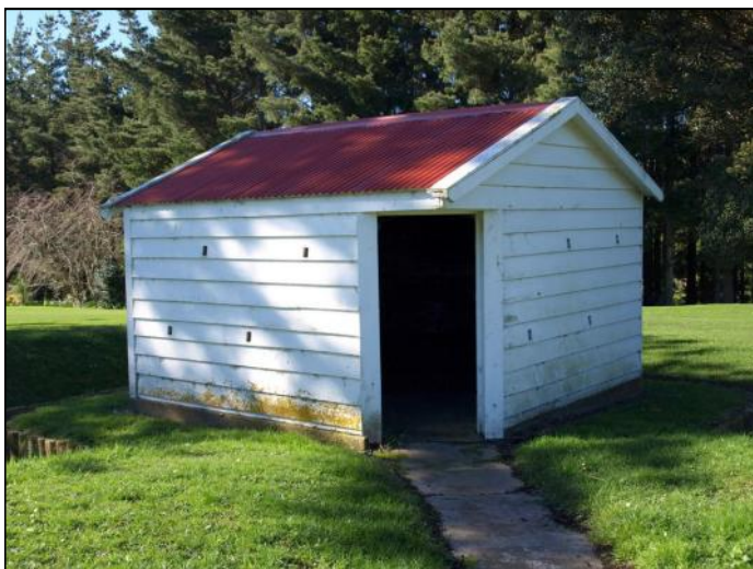
Block house with loop holes evident
