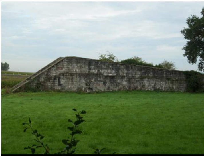
Hazebrouck - The concrete protective walls of the launch ramp.
