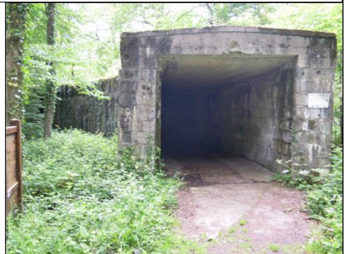
Hazebrouck - The curved entrance to the "hockey stick" building where V1 rockets were stored one behind the other prior to having their wings attached.
