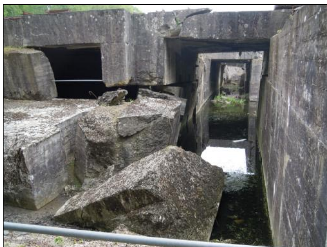
Damage to the railway station caused by Tall Boy bombs. The roof section shown would be 1m thick giving an indication of the size of the concrete blocks in the foreground.
