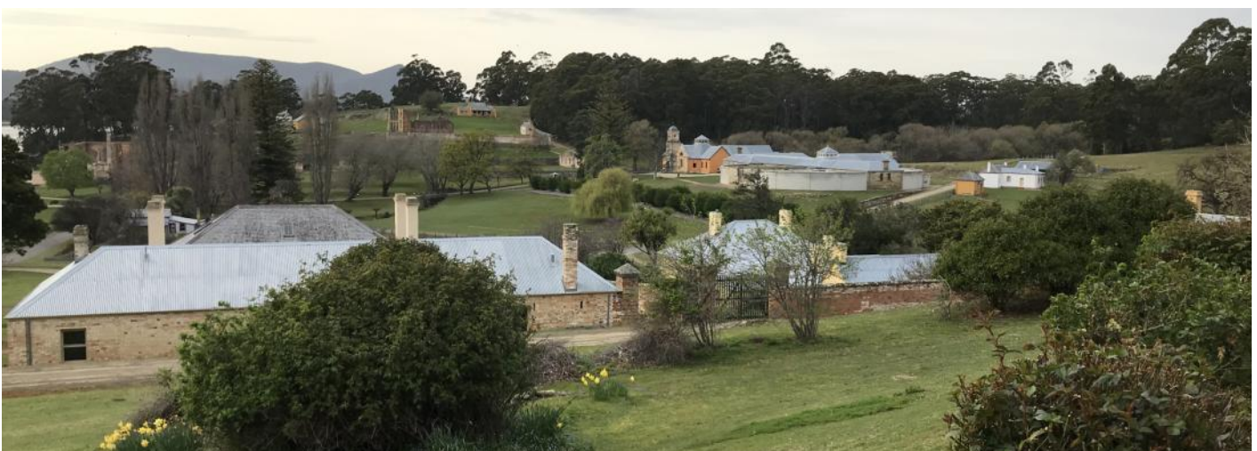
The houses in the foreground were for civilian staff - Chaplain, Medical Officer, Magistrate. The circular white structure right of centre is the Solitary Prison
